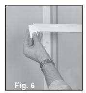
1 Slide corner backing angles into header casing.
