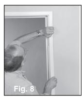
3 Slide jamb casing over corner backing angles. Align with jamb clips then snap on casing.
